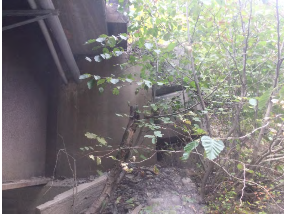
Photo 17 Right upstream wing wall
