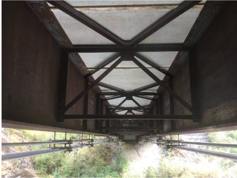
Photo 11 Underside of deck condition
