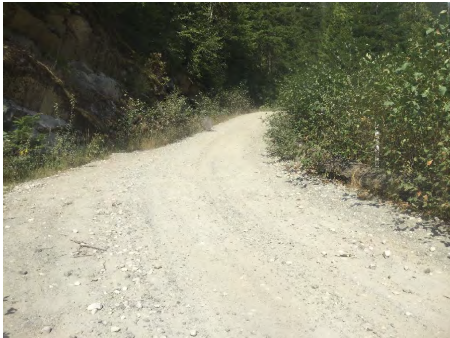
Photo 8 Right approach looking away from bridge
