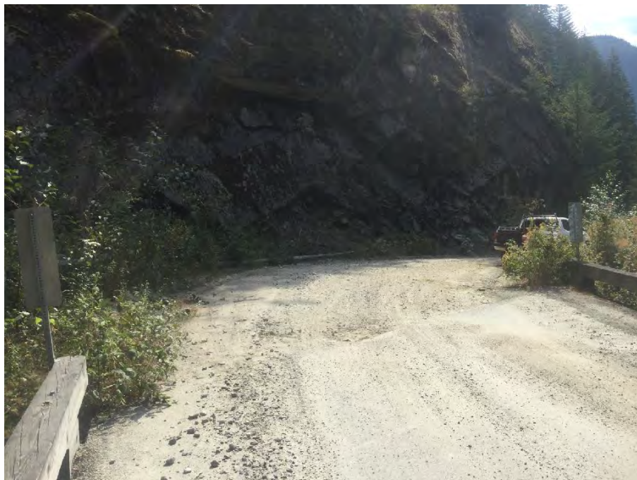
Photo 6 Left approach looking away from bridge
