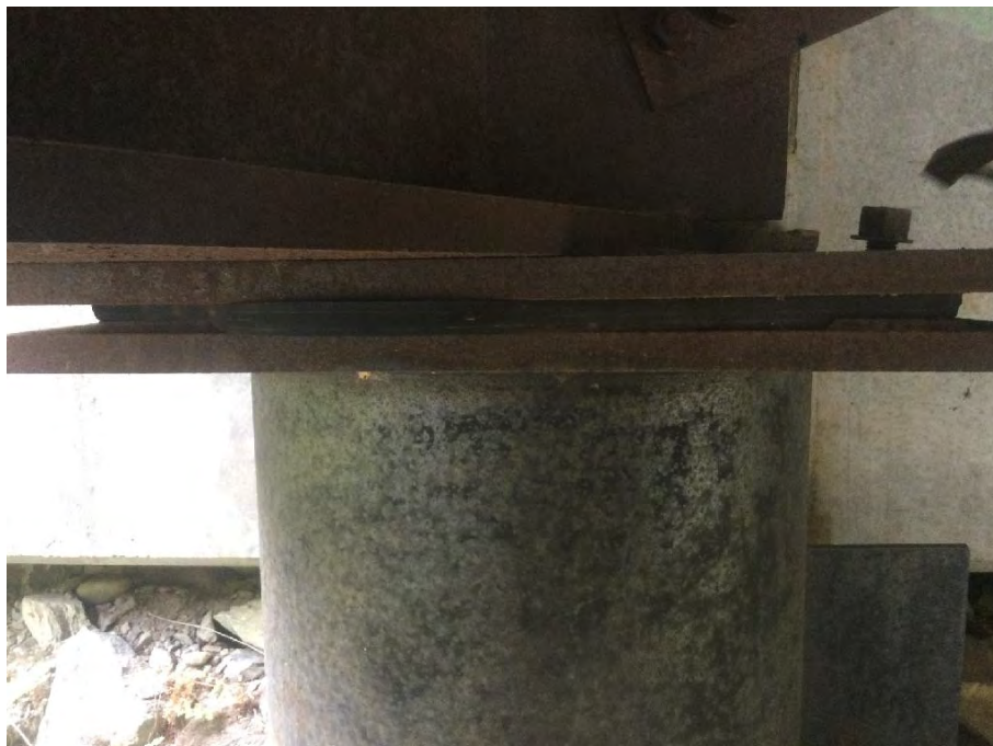
Photo 22 Typical bearing condition
