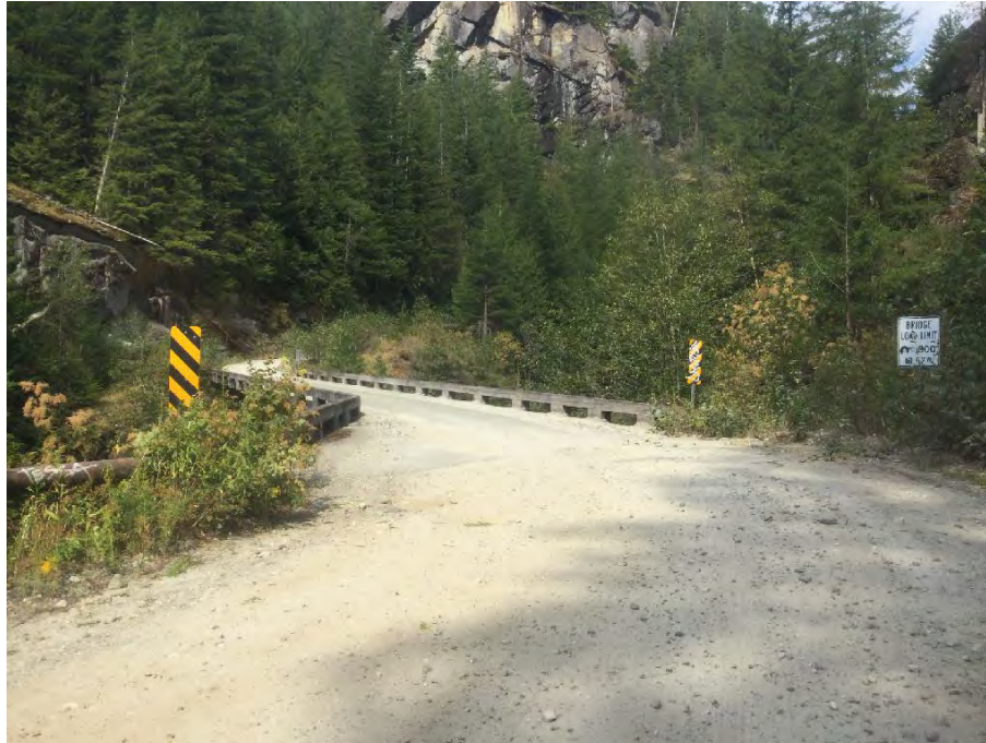
Photo 5 Left approach looking towards bridge
