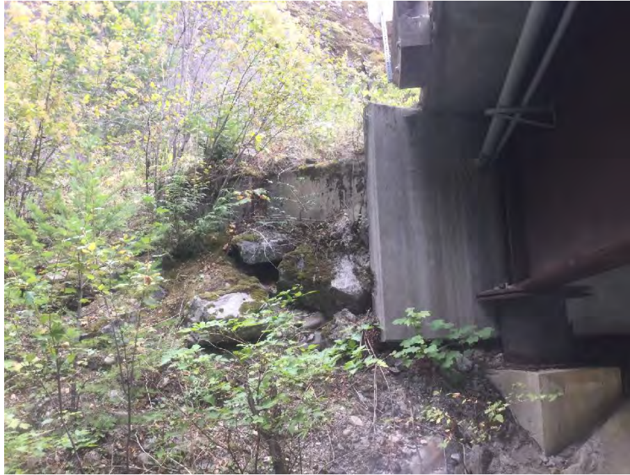
Photo 15 Left upstream wing wall
