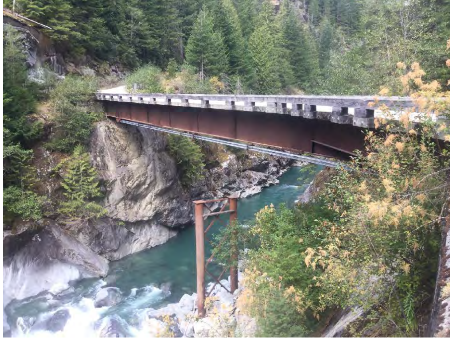
Photo 1 Bridge elevation from downstream
