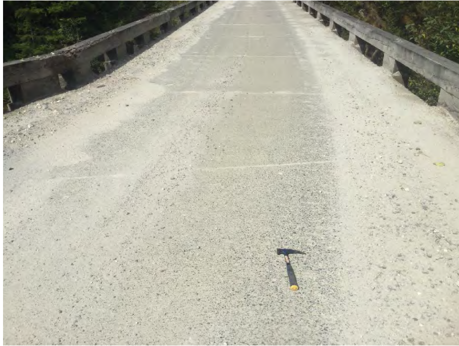
Photo 9 General deck condition
