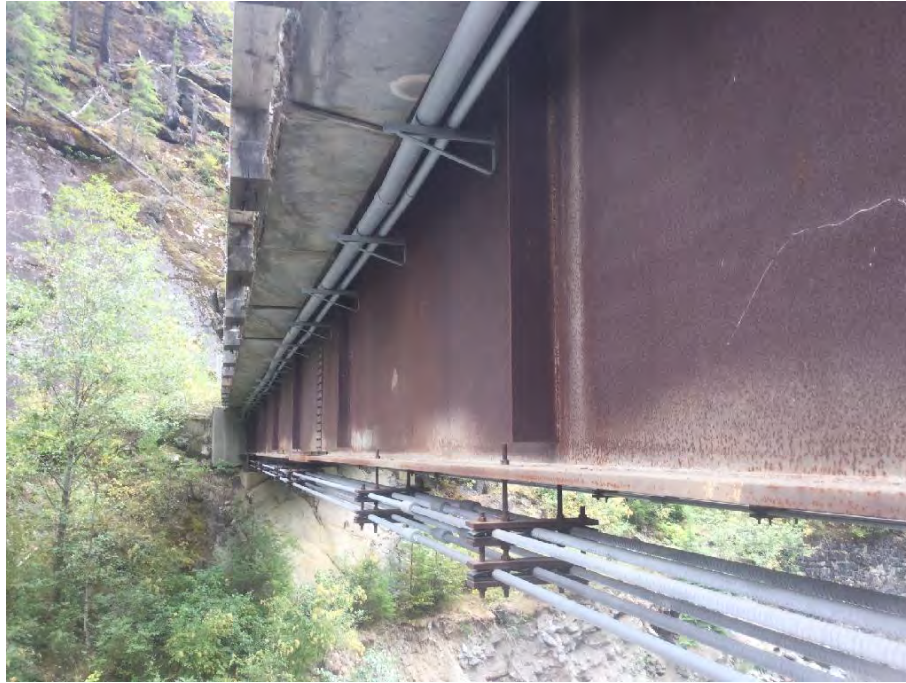
Photo 19 Typical girder condition
