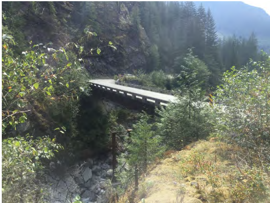
Photo 2 Bridge elevation from upstream
