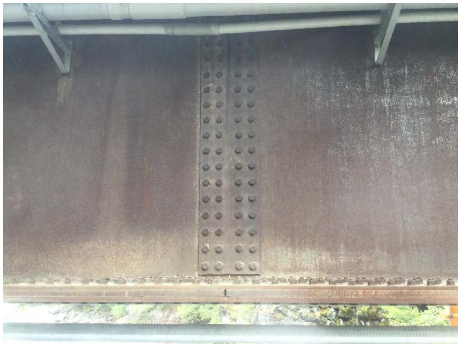
Photo 20 Typical splice condition
