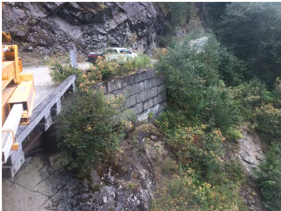
Photo 16 Left downstream wing wall
