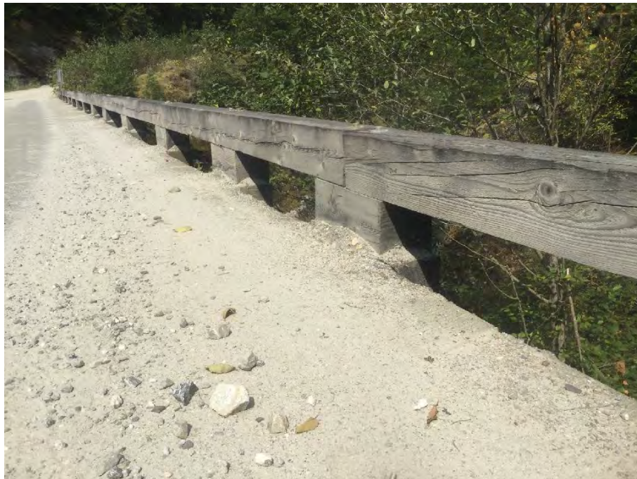
Photo 10 General railing condition
