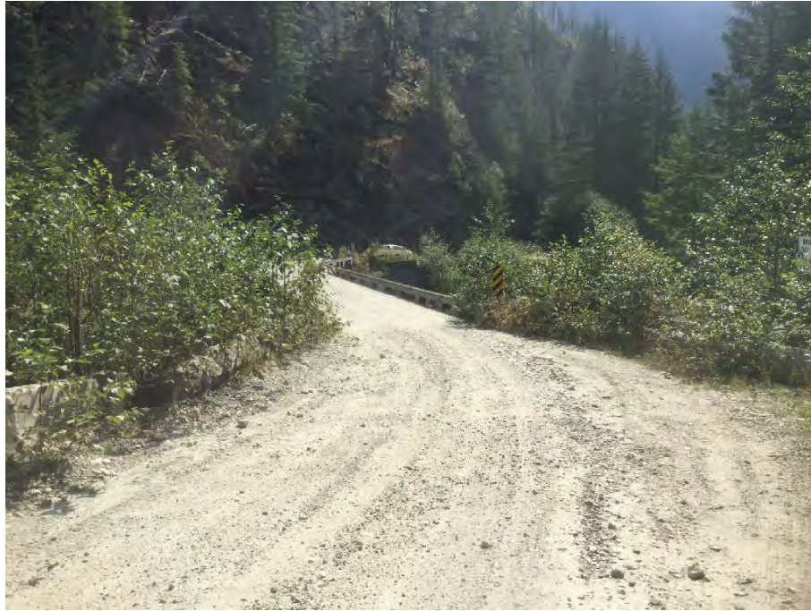
Photo 7 Right approach looking towards bridge
