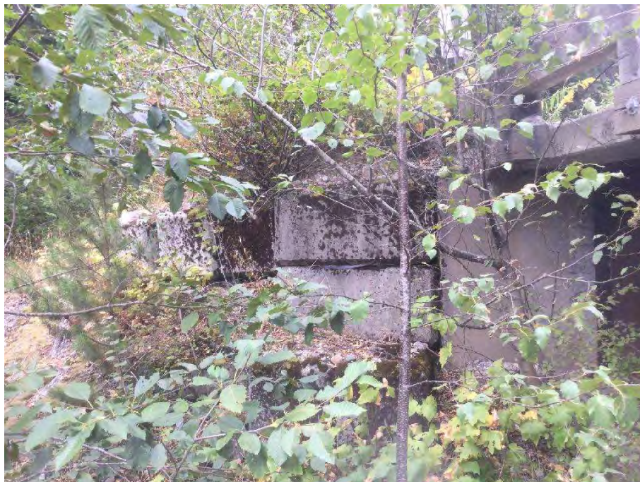
Photo 18 Right downstream wing wall
